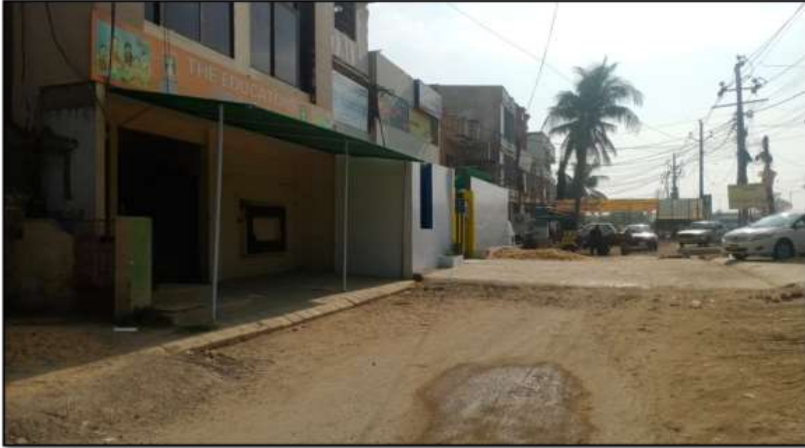
Nullah encroached in front of White House Scheme 33, District Malir
